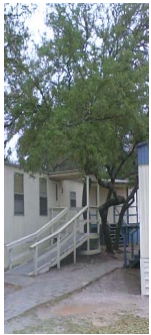
Our portable classrooms
